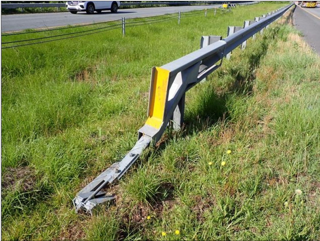
northeast guardrail termination
