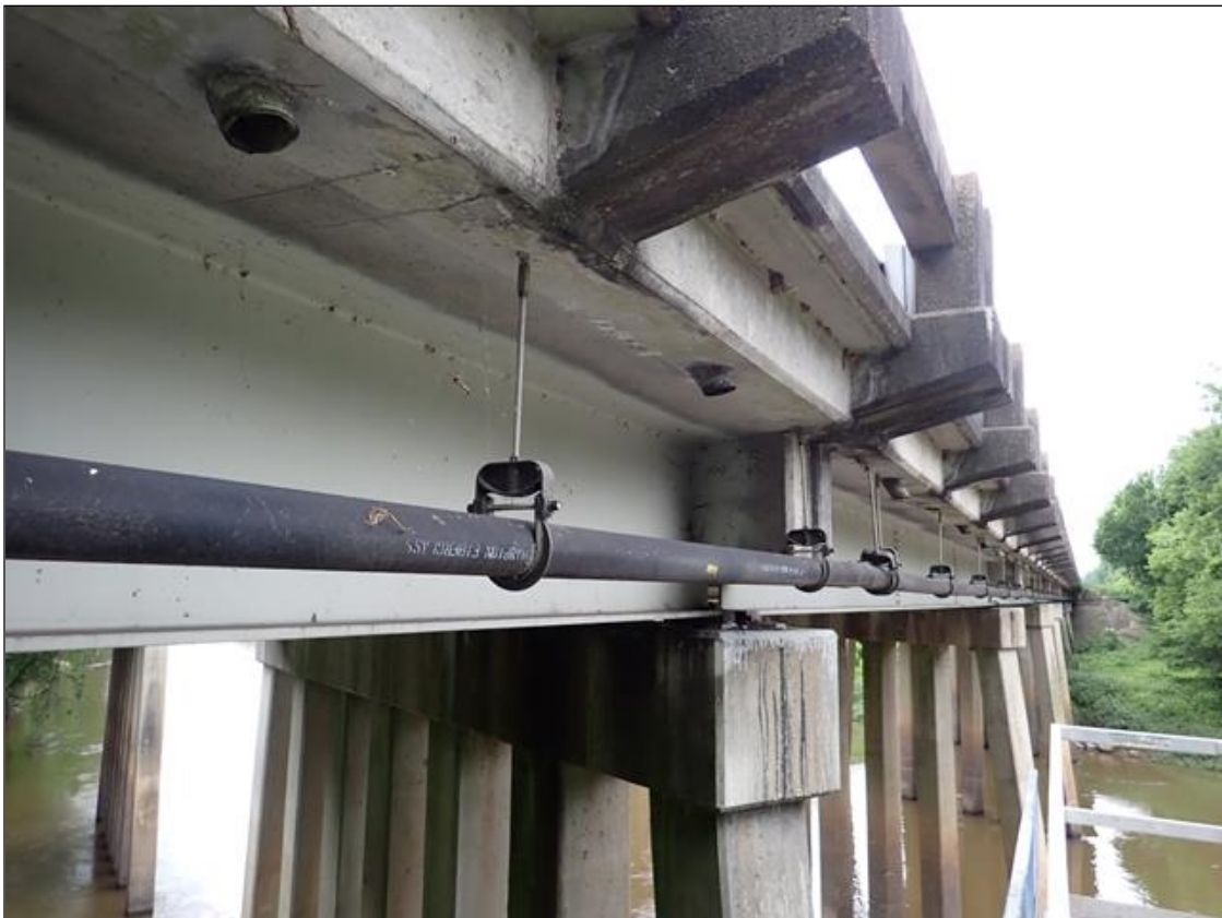
along west fascia, utility pipe (4 inch diameter)
