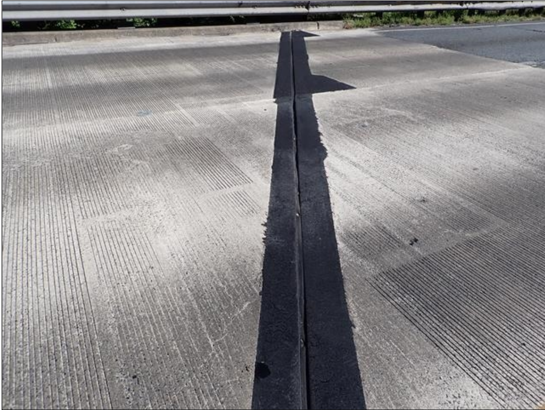
end bent 2 joint
