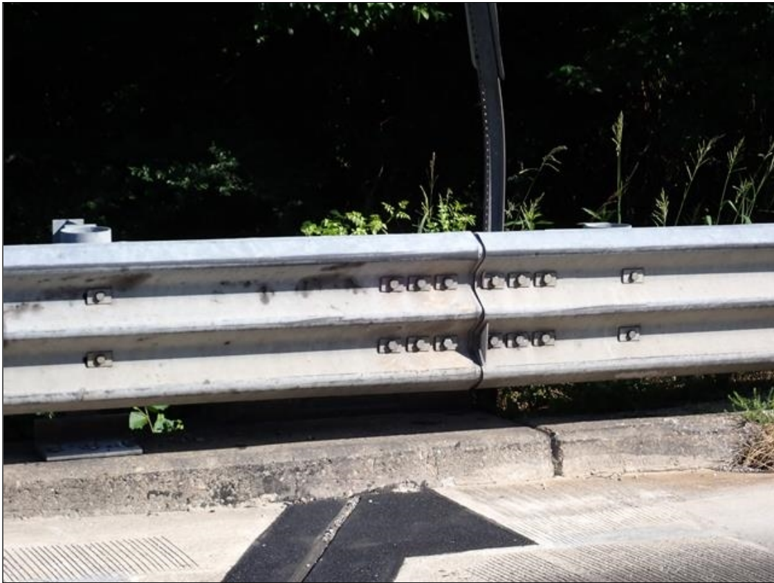
northwest guardrail attachment
