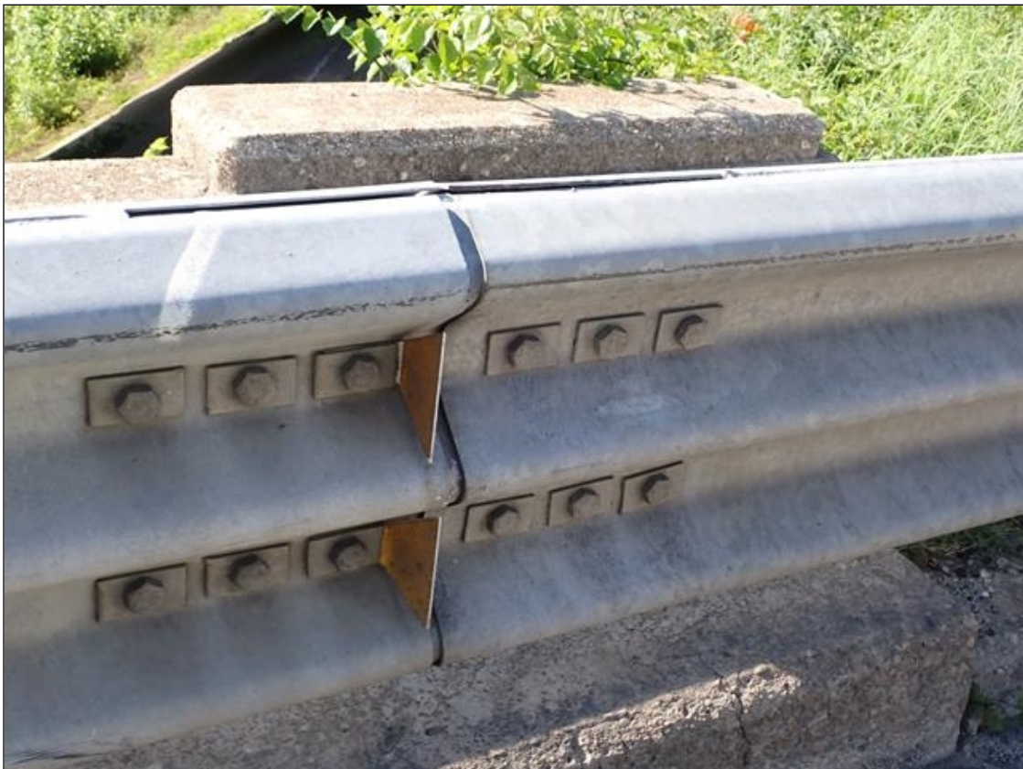
southeast guardrail attachment
