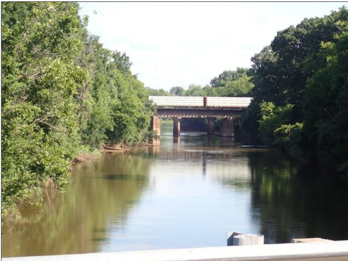
upstream looking west
