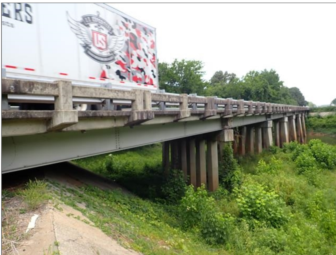
east profile looking west
