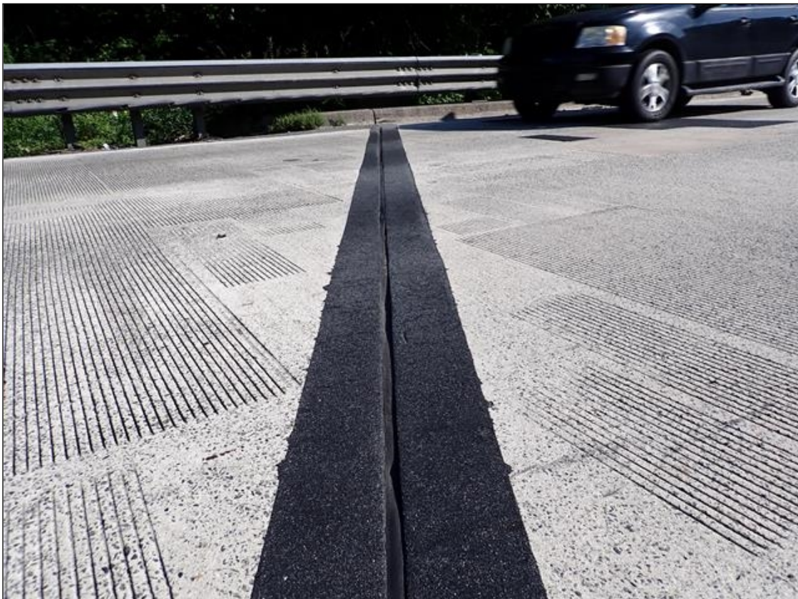
end bent 1 joint
