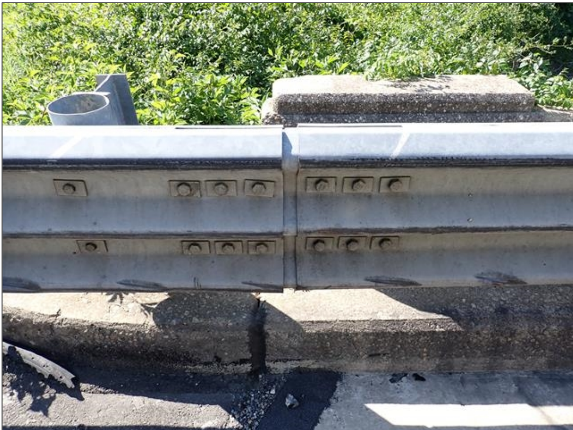
northeast guardrail attachment
