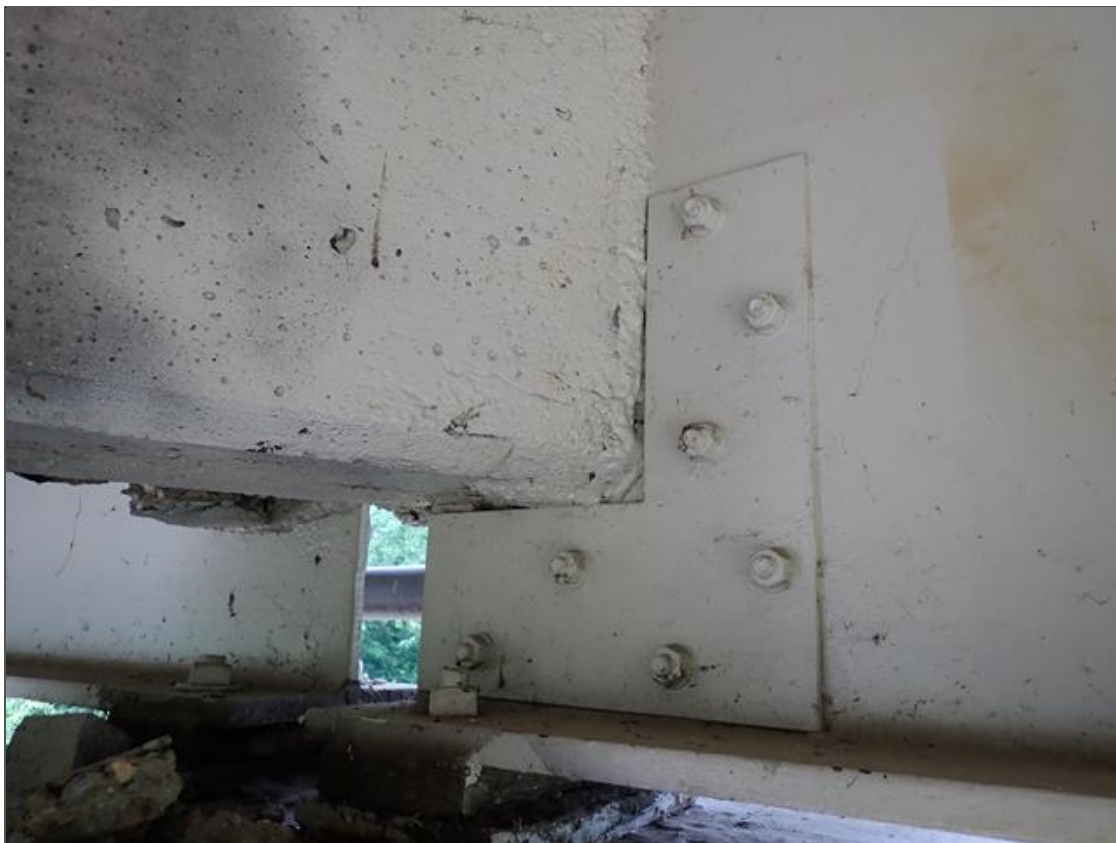
Span 5 Beam 1: at bent 4, web repair plate, (3/8 inch thick x 15.5 inch x 17 3/4 inch)
