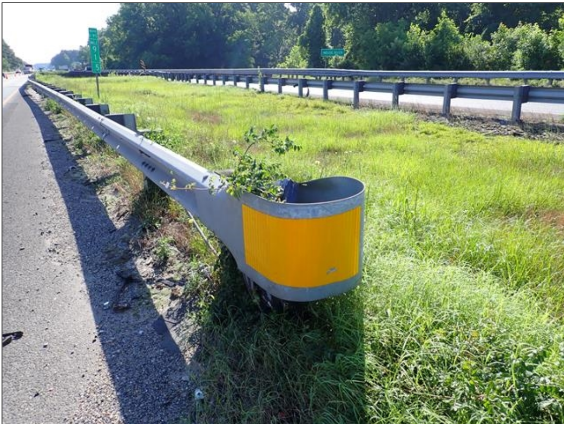
southeast guardrail termination
