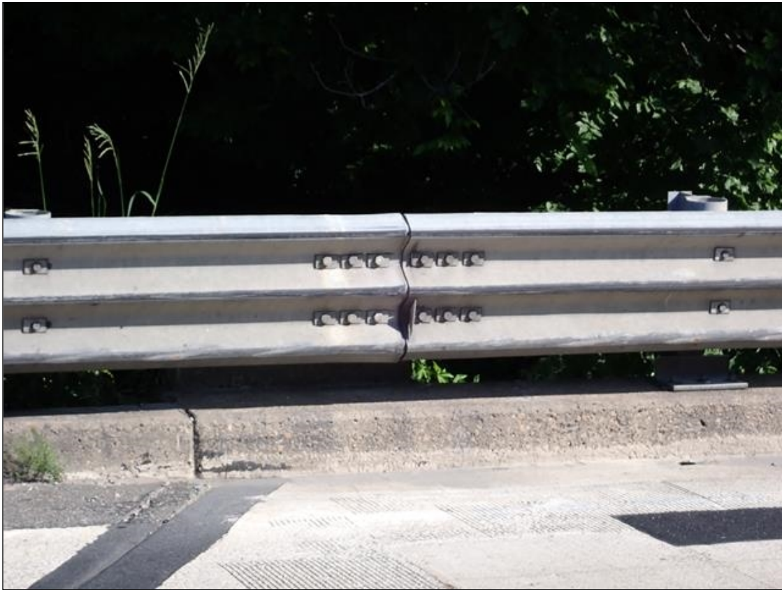
southwest guardrail attachment
