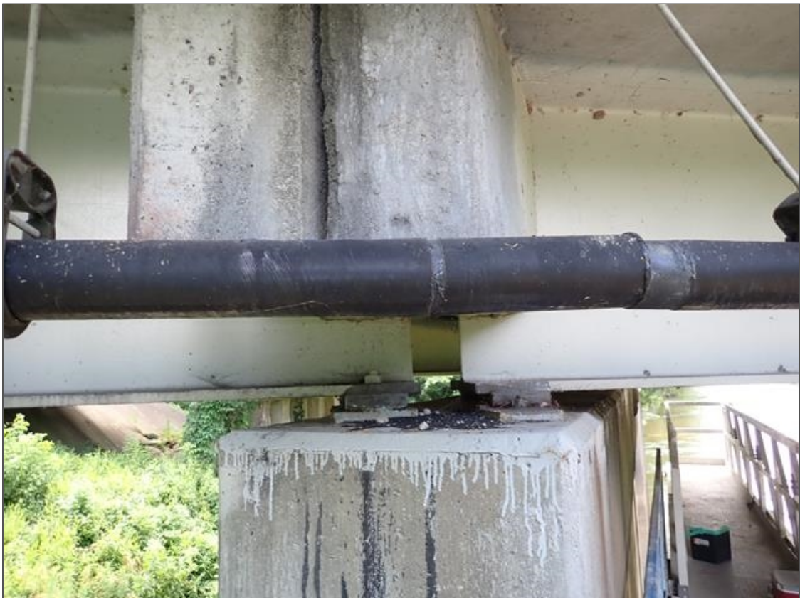
beams over bent
