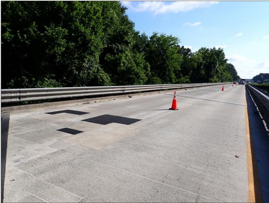
left bridge rail
