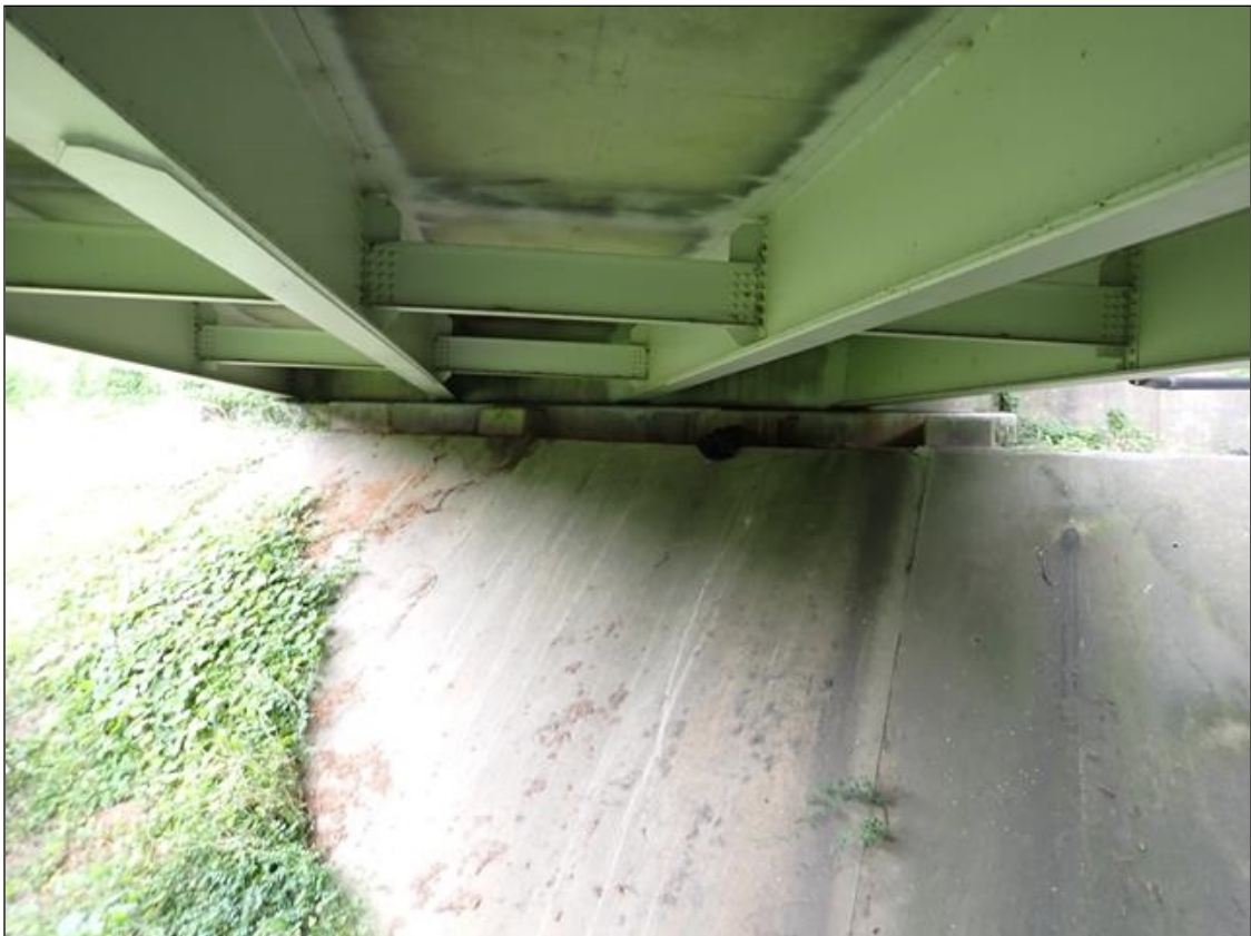
end bent 1 and slope protection
