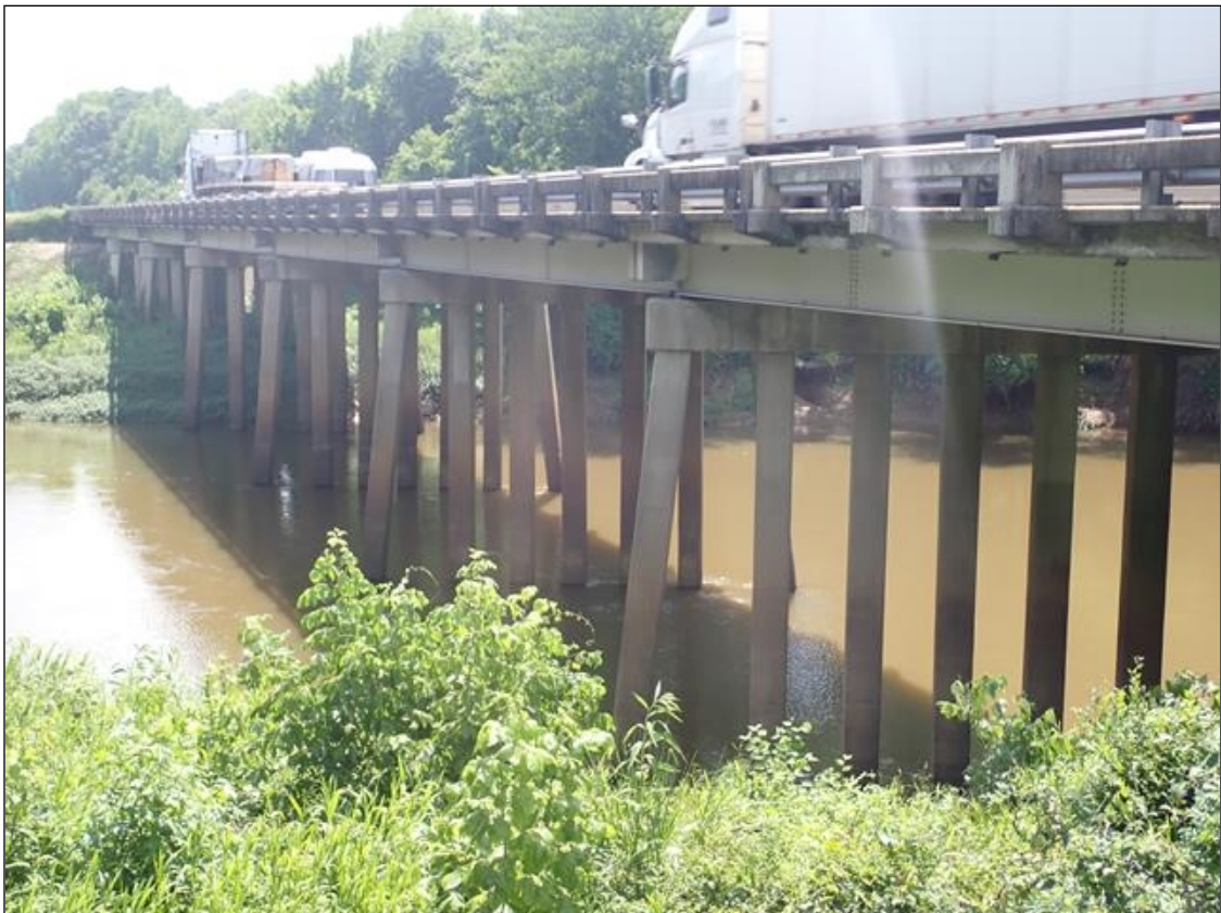
downstream profile looking west
