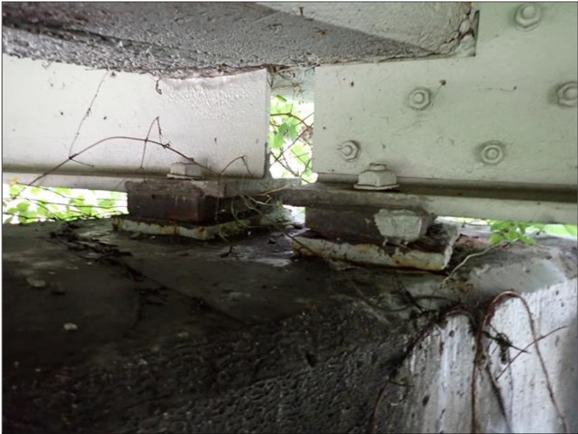
interior bearing assembly
