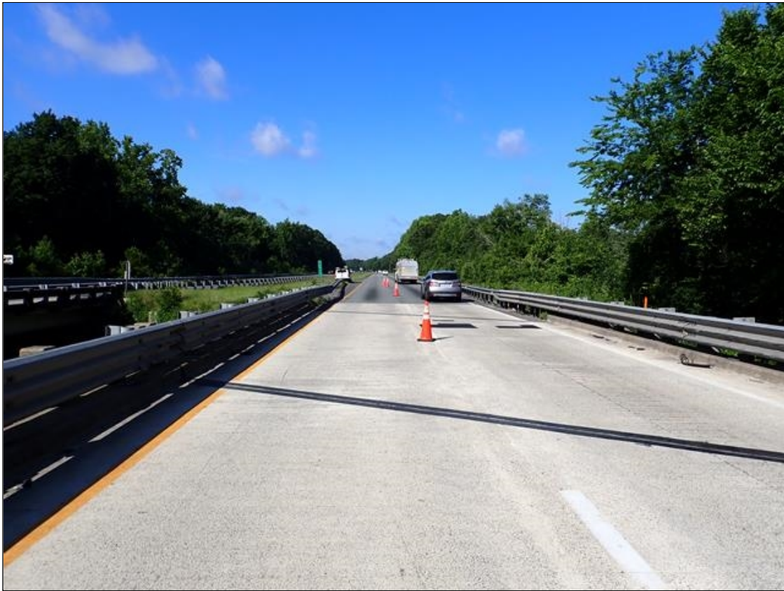
south approach looking south
