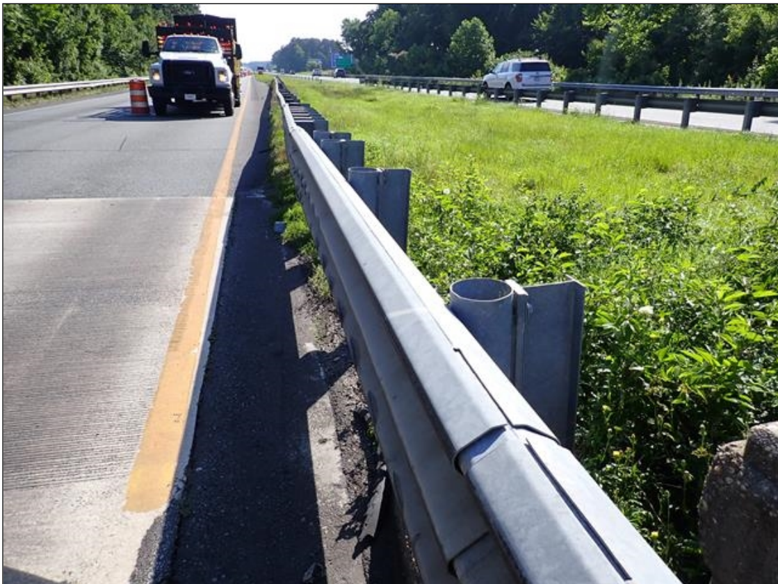
northeast guardrail transition
