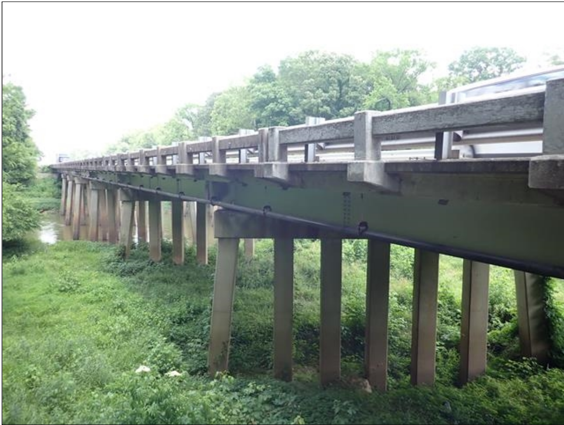
west profile looking east
