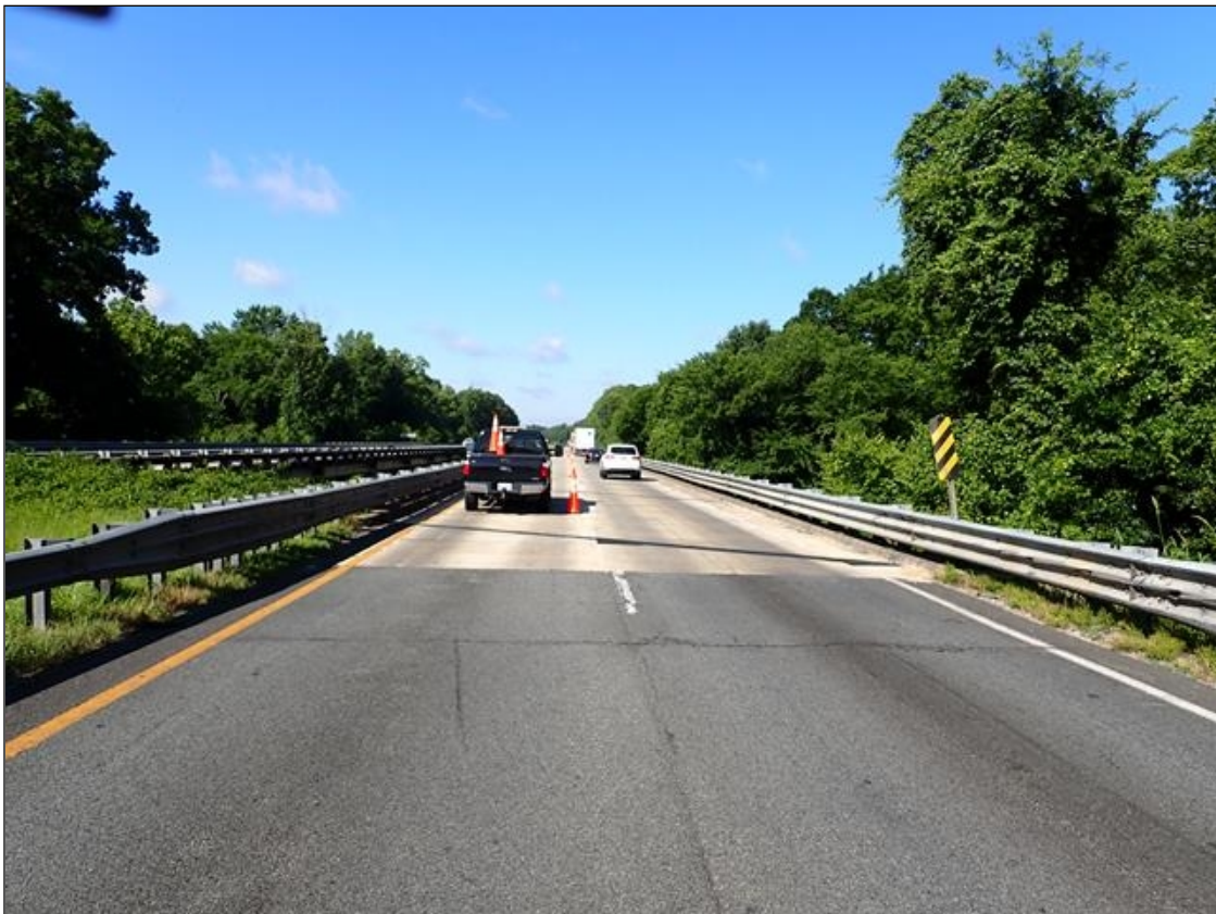
north approach looking north
