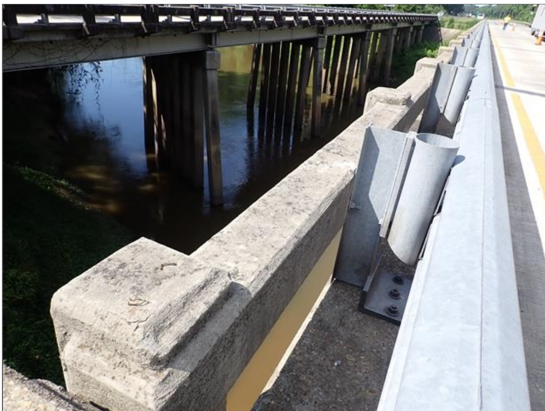
Span 7 Right Bridge Rail: AT MIDSPAN, 15 FEET LONG SECTION OF CONCRETE RAIL HAS BEEN REPLACED
